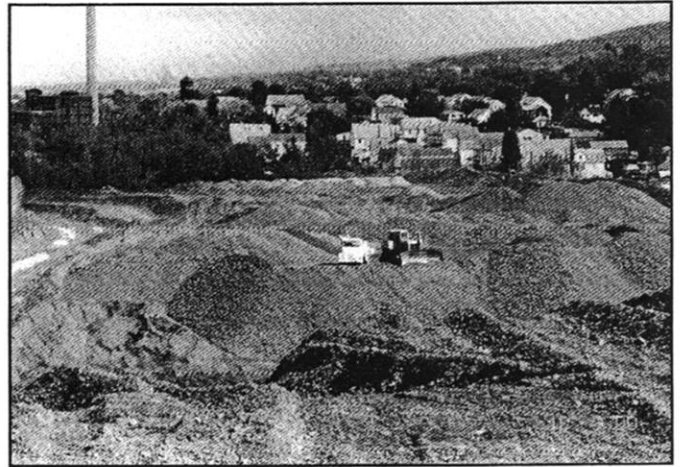
The Preston Bank reclamation project was funded through a $750,000 Growing Greener Grant EC received in 2000. Here, piles of culm, mine rock and other mining wastes are being leveled, in order to make the site reusable for future development.
