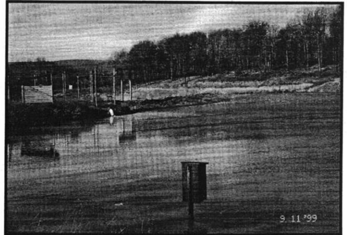
EC's Phase II Wetland site has been treating mine drainage from the Askam Borehole since the Spring of 1999. Recent water quality testing shows that this wetland is removing more than 96 percent of the iron that is present in the water when it first enters the site.
