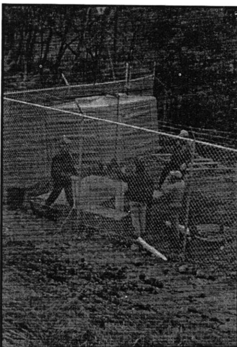
Workers installed the Maxistripper last month. It adds oxygen to the water as it enters the wetland, making the iron particles heavier and causing them to fall to the bottom.
