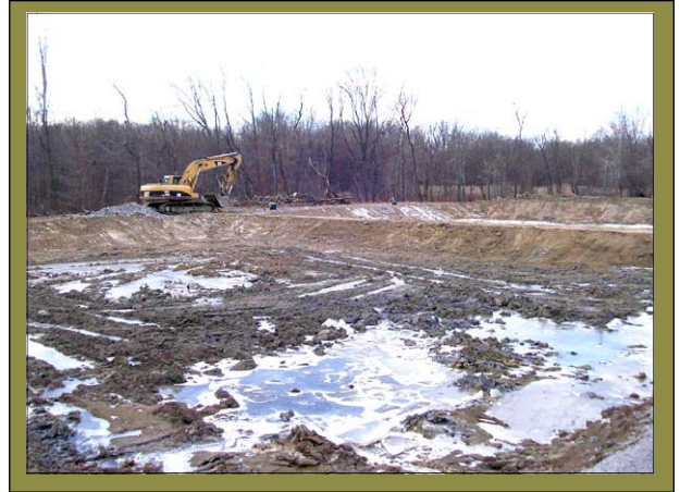
Pictured above are the two settling ponds for the Espy Wetlands AMD Enhancement Project, with a berm dividing the two ponds.
