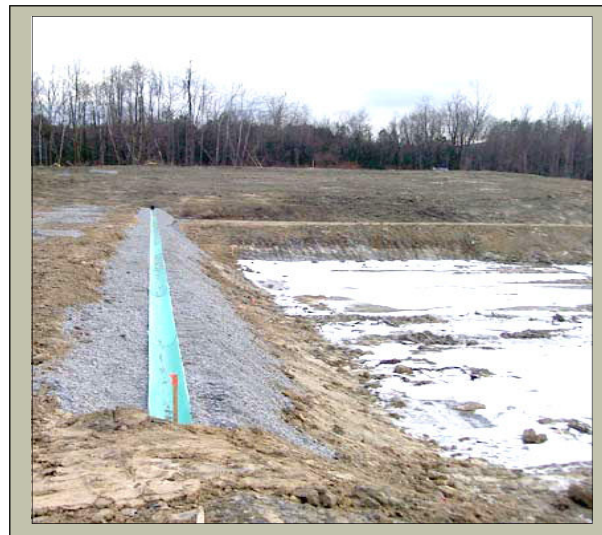
The green piping will serve as an inlet for water from the Espy Discharge into the two settling ponds. Once in the settling ponds, iron deposits will sink to the pond bottom, thus clearing the water.
