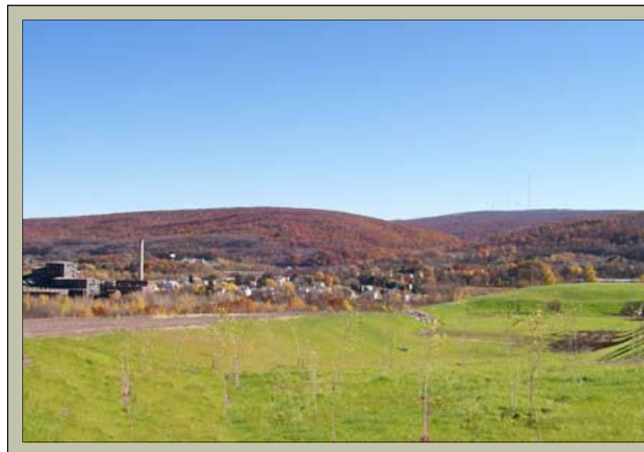
The reclaimed Huber IV site will remove the culm banks and pits from the site, as shown by this completed section.
