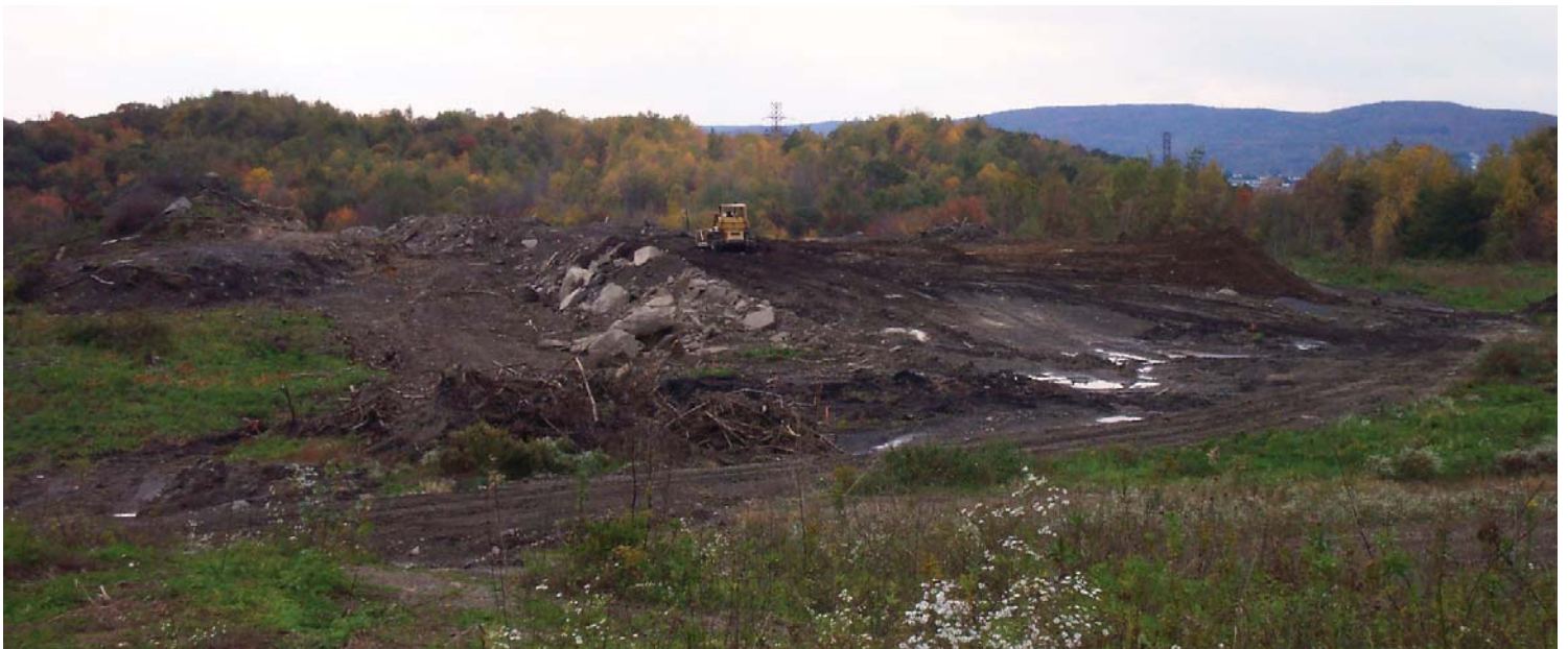
Recreational Park ~ With the initial portion of the park completed, work on the Greater Hanover Area Recreation Park continues with Phases II and III.
