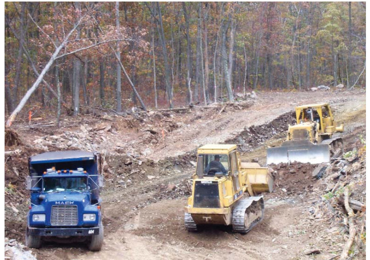
Nuangola Residential Development ~ Workers move earth as they excavate the road for the new Woodland Acres development in Nuangola.
