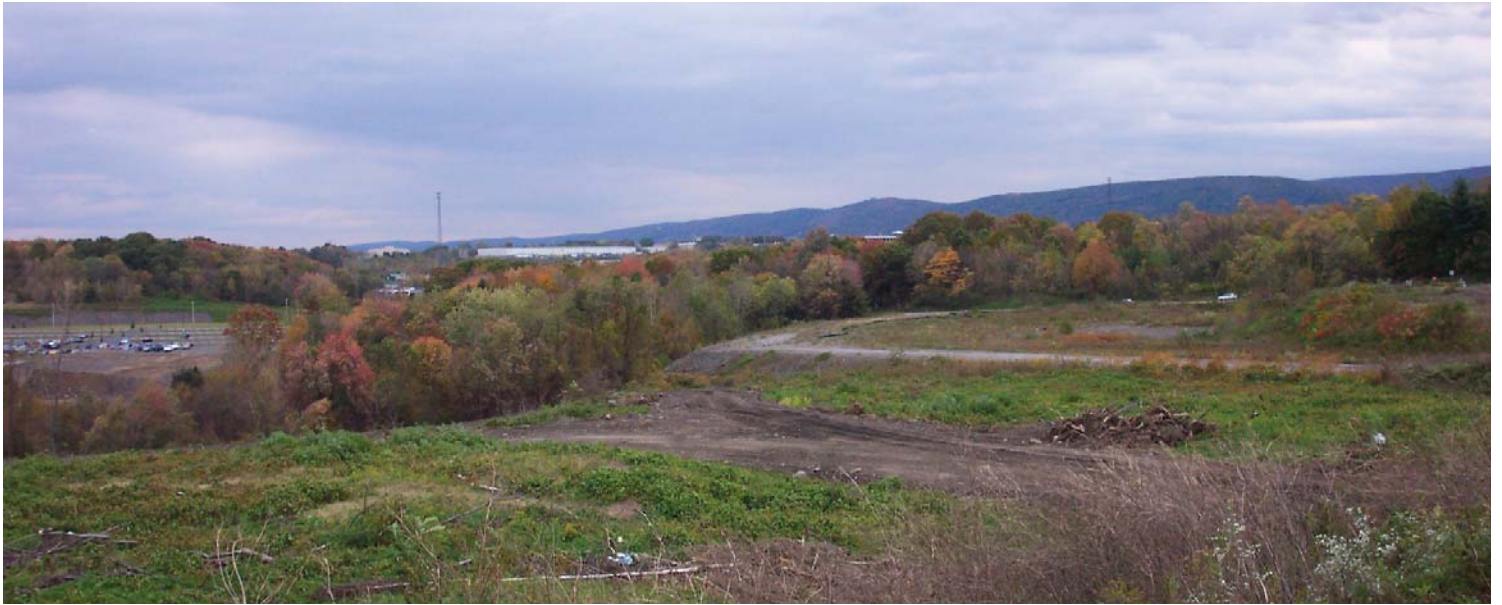
Landfill ~ Reclamation of the former Luzerne County Flood Debris Landfill is well underway, with much of the remnants of the Agnes Flood disappearing from sight.
